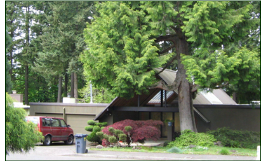
Striking post-and-beam home with an internal orientation, open floor plan and expansive interior glass provides private views of nature.
